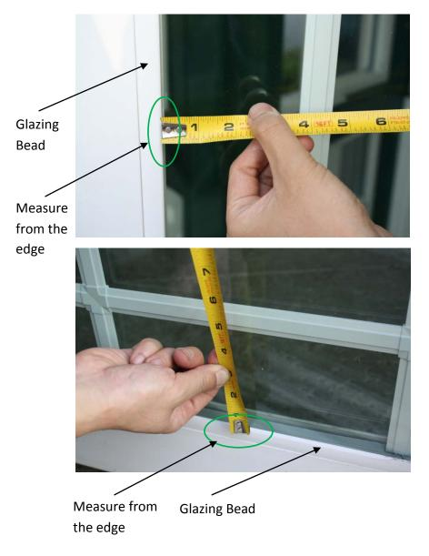
For Example, the size you measured is 48x52, then the actual size of the glass to order is  $48\frac{7}{8} \times 52\frac{7}{8}$ °.
